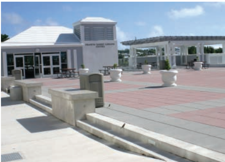
The spacious new piazza atop the Gosling Centre
