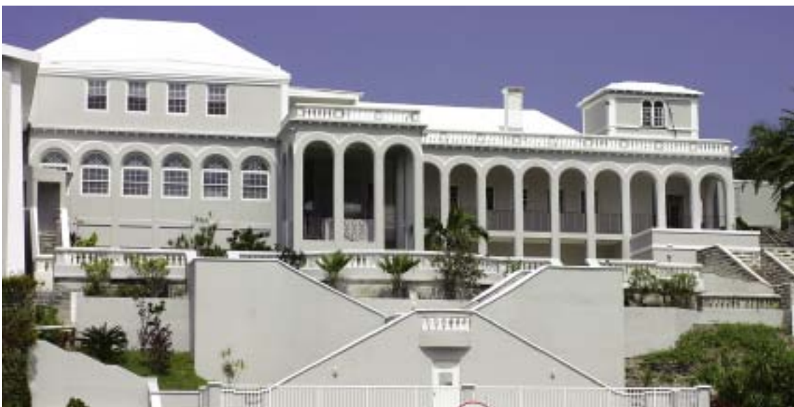
New look: Woodlands and Upper Primary buildings with their new coat of paint
